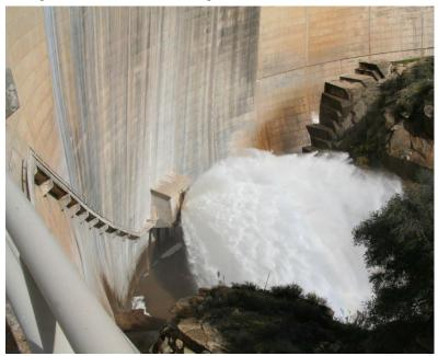
The outlet works at Loveland have two valves that are 78 years old and in need of replacement. In addition, a portion of the concrete stairway to the valve house has deteriorated and needs to be rebuilt.
