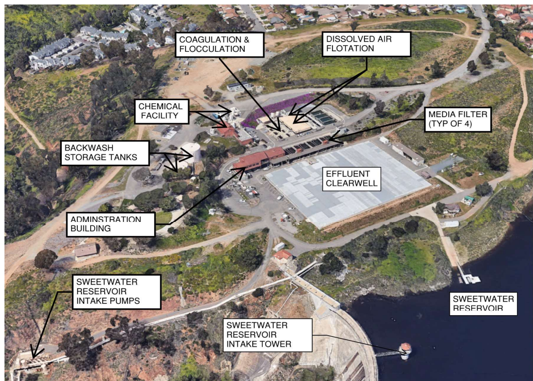
Figure 1.1 Overview of Perdue WTP Existing Facilities
