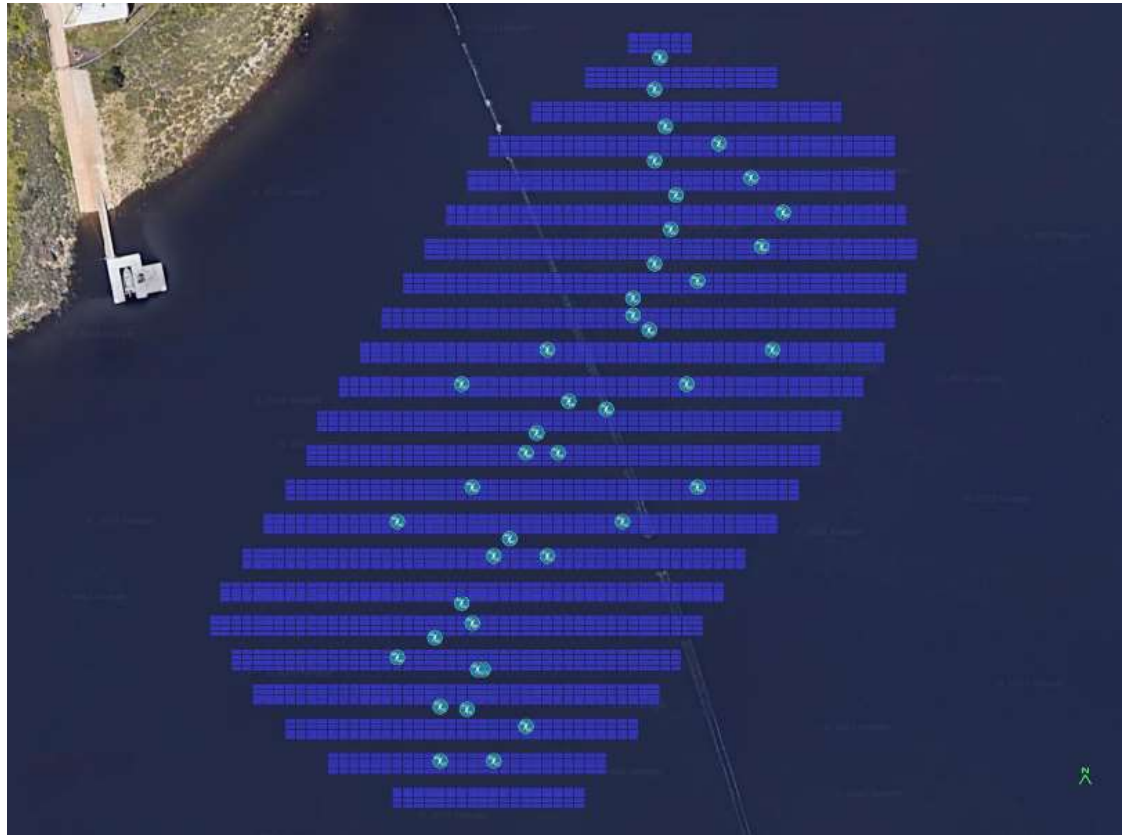
Figure 5.22 Floating Solar Array
