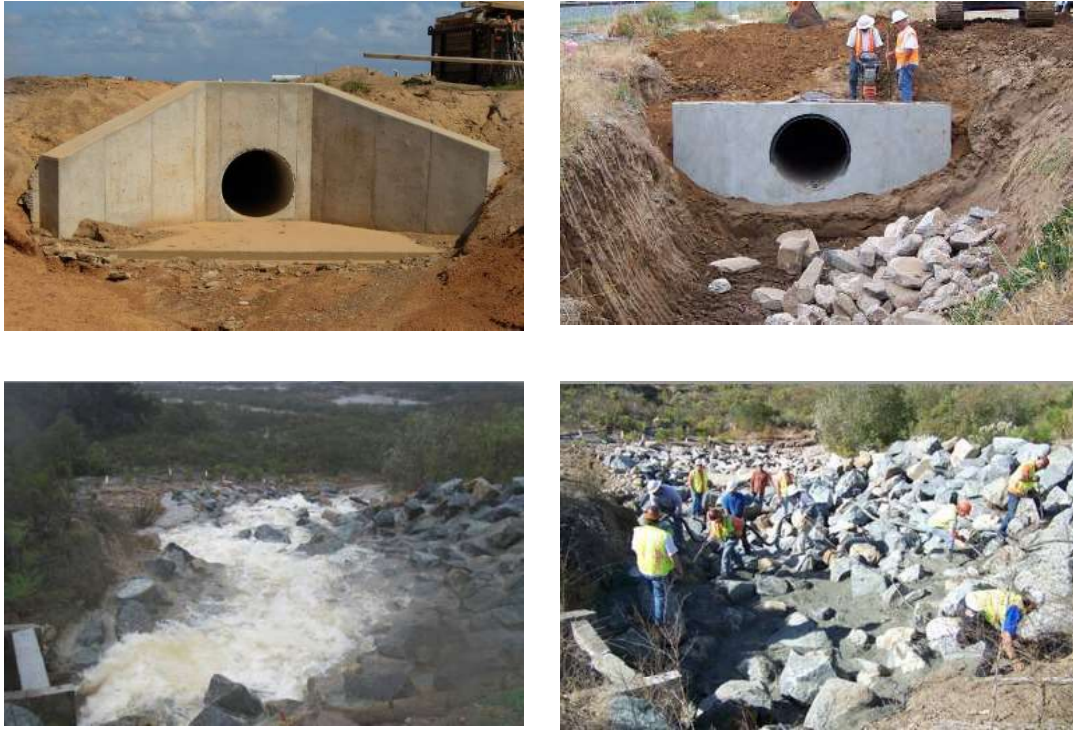
Figure 3.7 Typical Outlet Headwalls and Grouted Riprap Channel
