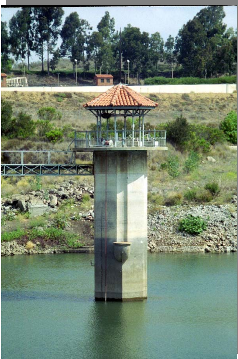
Photo 3 – Outlet tower as viewed from left abutment (taken June 3, 2002).
