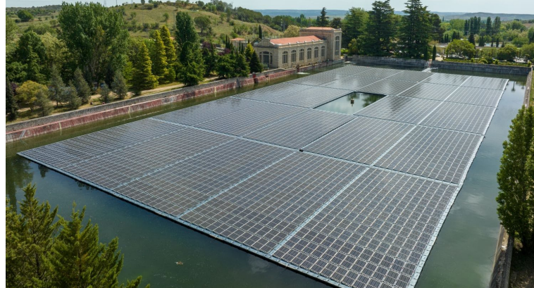
1.7 MW solar array at Canal Isabel II's Torrelaguna Plant (Spain) - 2023
