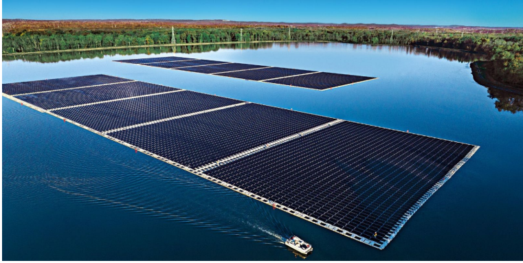
8.9 MW solar array covers 17 acres of the Canoe Brook reservoir in Short Hills, New Jersey - 2023
