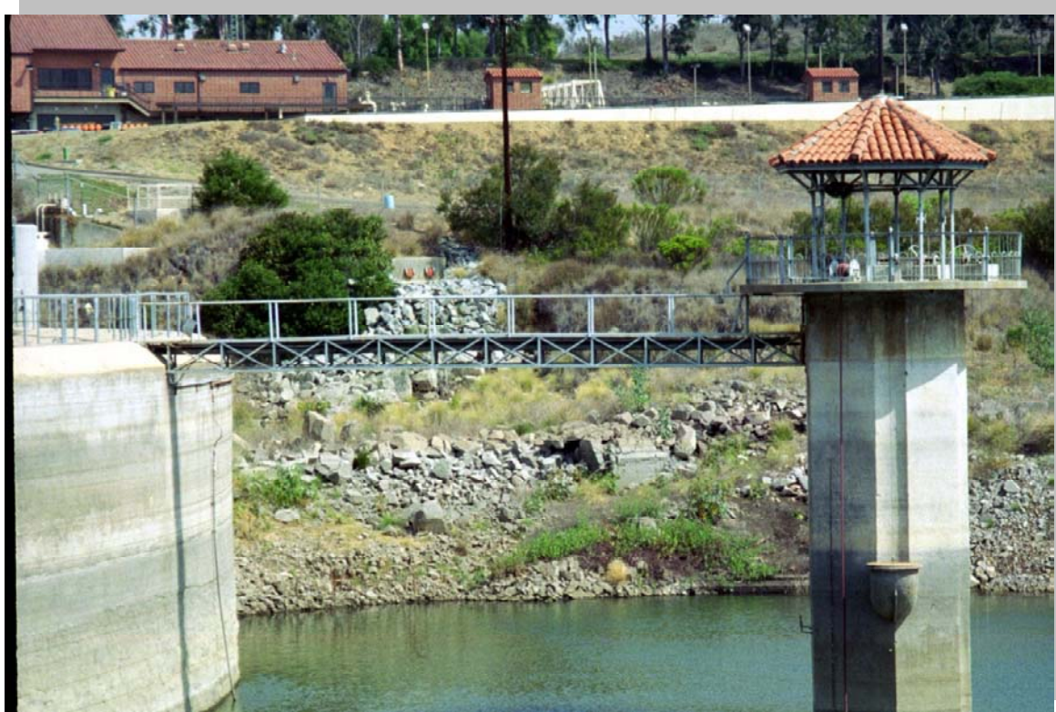
Photo 2 – Outlet tower and bridge as viewed from left abutment (taken June 3, 2002).
