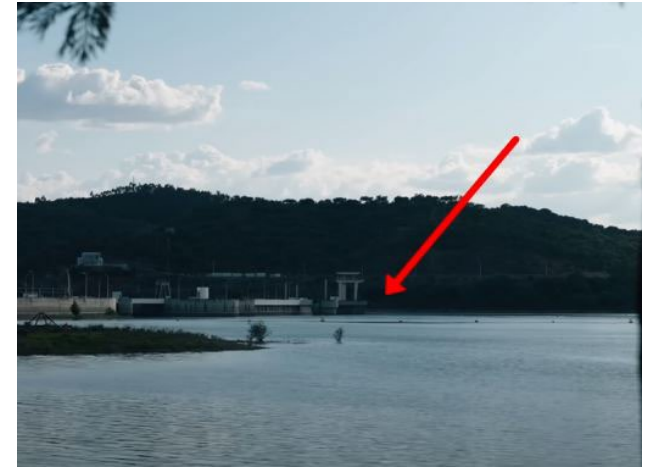
Example of shoreline view of floating solar
